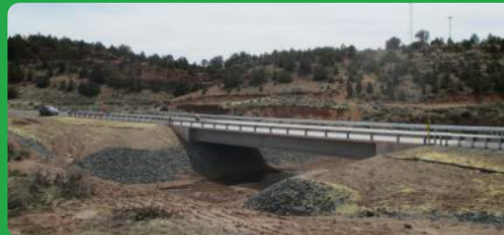
Location: Kinlicee, AZ Client: BIA Project: Cast-in-Place Bridge w/ Erosion Protection
